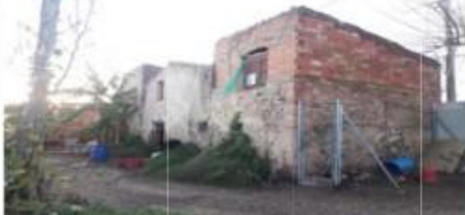
1 Mas i coberts existent a rehabilitar
